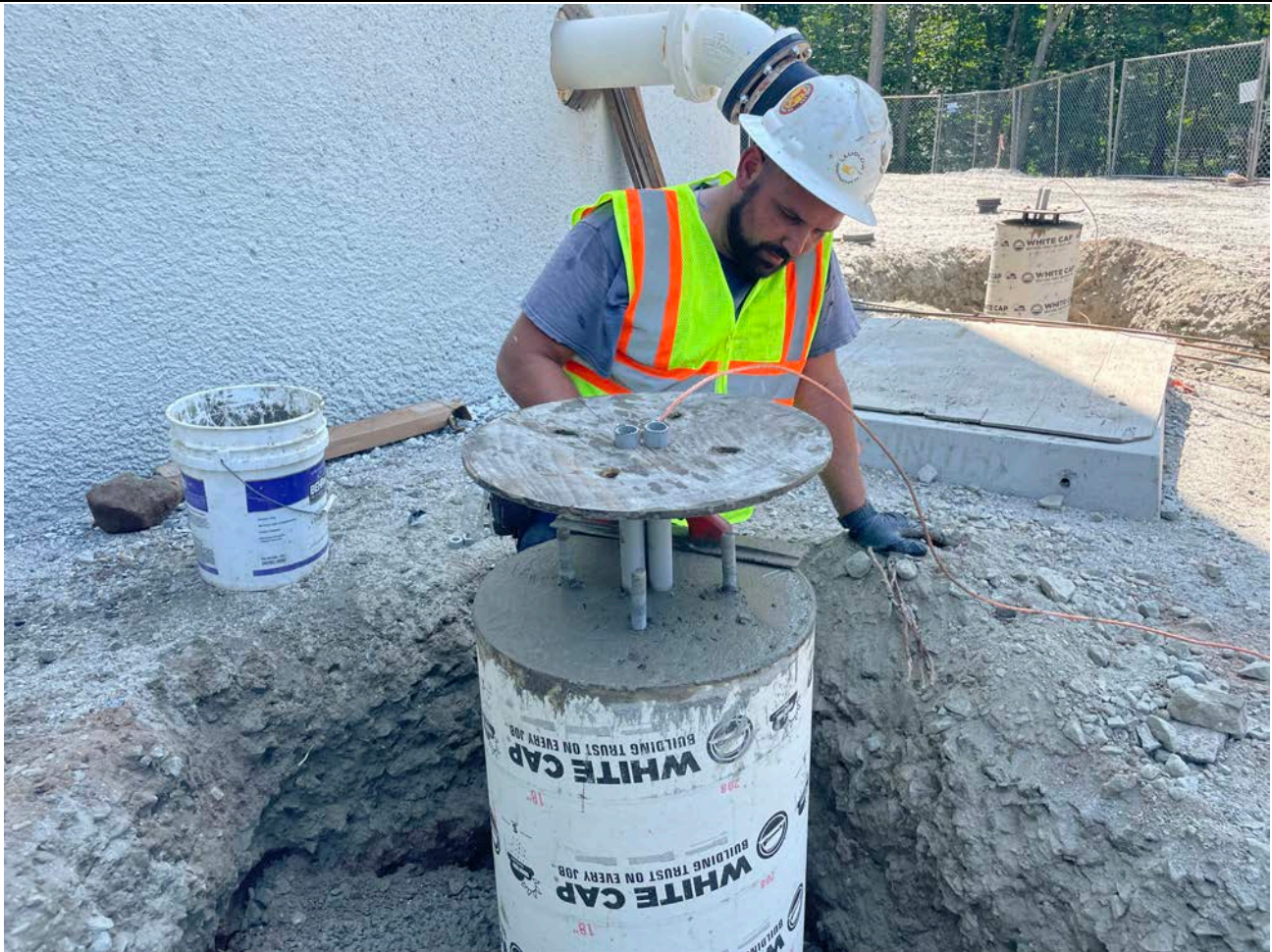
Picture 2: Ludlow leveling concrete that was placed into the sonotubes for the light pole bases at the water tank work zone located east of the Shared Access Driveway in Middletown today. View to the south.
