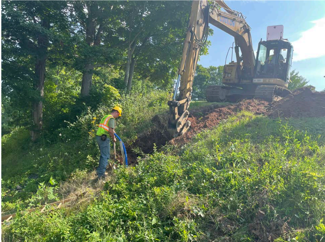
Picture 1: Ludlow excavating at 10 Johns Way next to Maple Avenue for the installation of a 1.5" copper water service line. View to the northeast.
