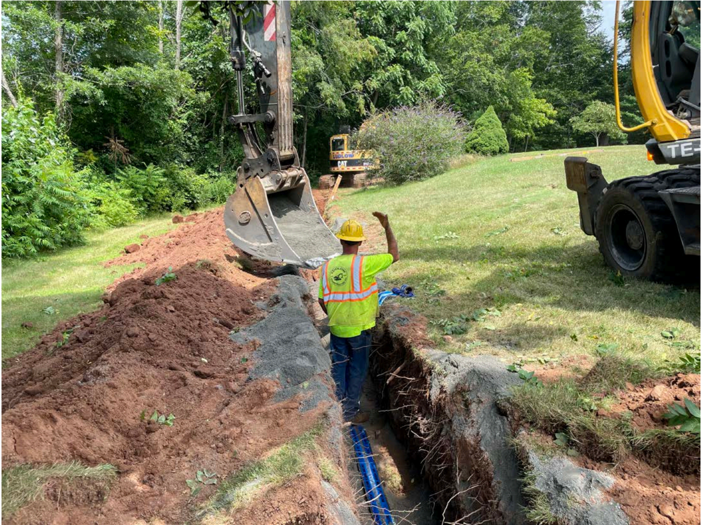
Picture 8: Ludlow placing sand and caution tape over 1.5" copper water service line at the residence located at 10 Johns Way, Durham. View to the north.
