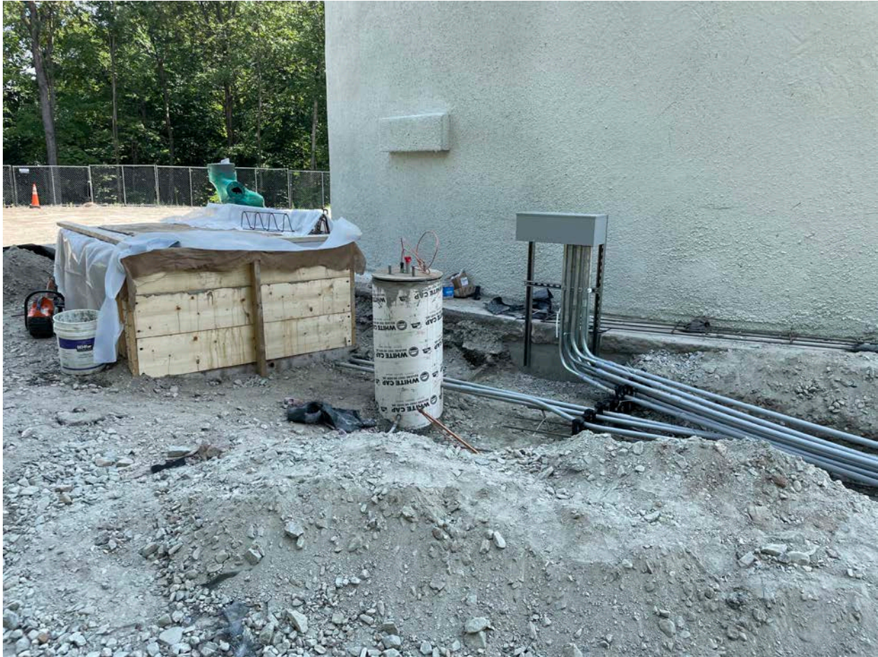
Picture 11: Overview of blower enclosure pad and conduit that has been installed on the northeast side of the water tank located east of the Shared Access Driveway. View to the south.
