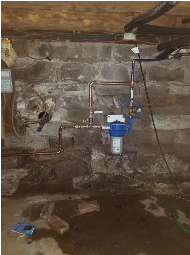
Picture 12: Final water service components that Fazzino Plumbing installed today at the residence located at 248 Main Street, Durham.
