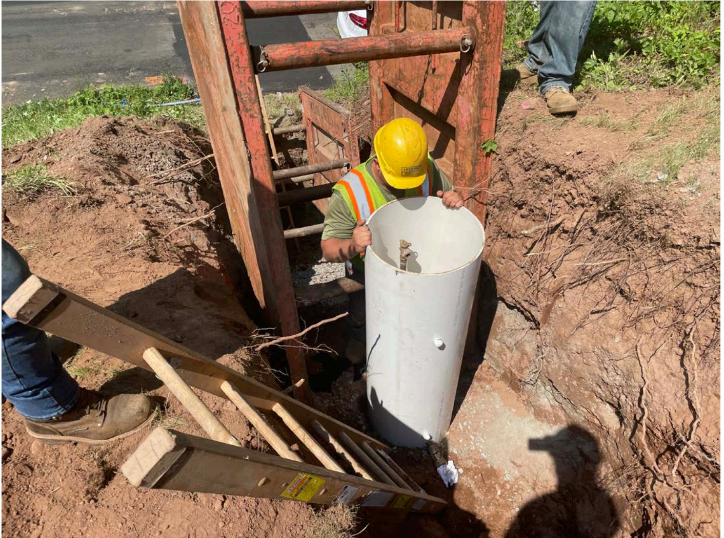
Picture 5: Ludlow setting meter pit in place in the trench that they excavated for the installation of a 1.5” copper water service line at the 10 Johns Way, Durham, residence. View to the northwest.
