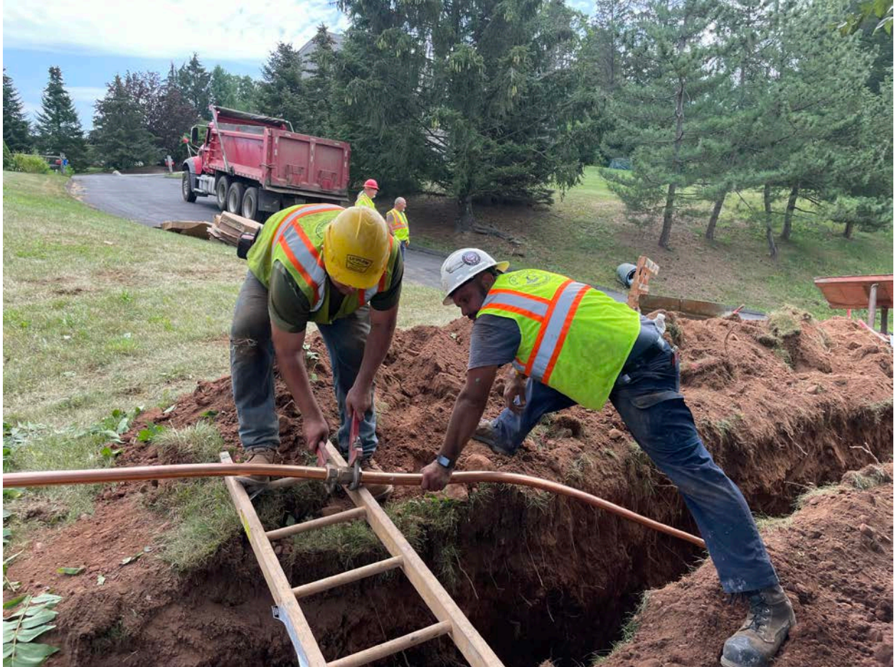
Picture 7: Ludlow joining two sections of 1.5" copper water service line at the residence located at 10 Johns Way, Durham. View to the east.
