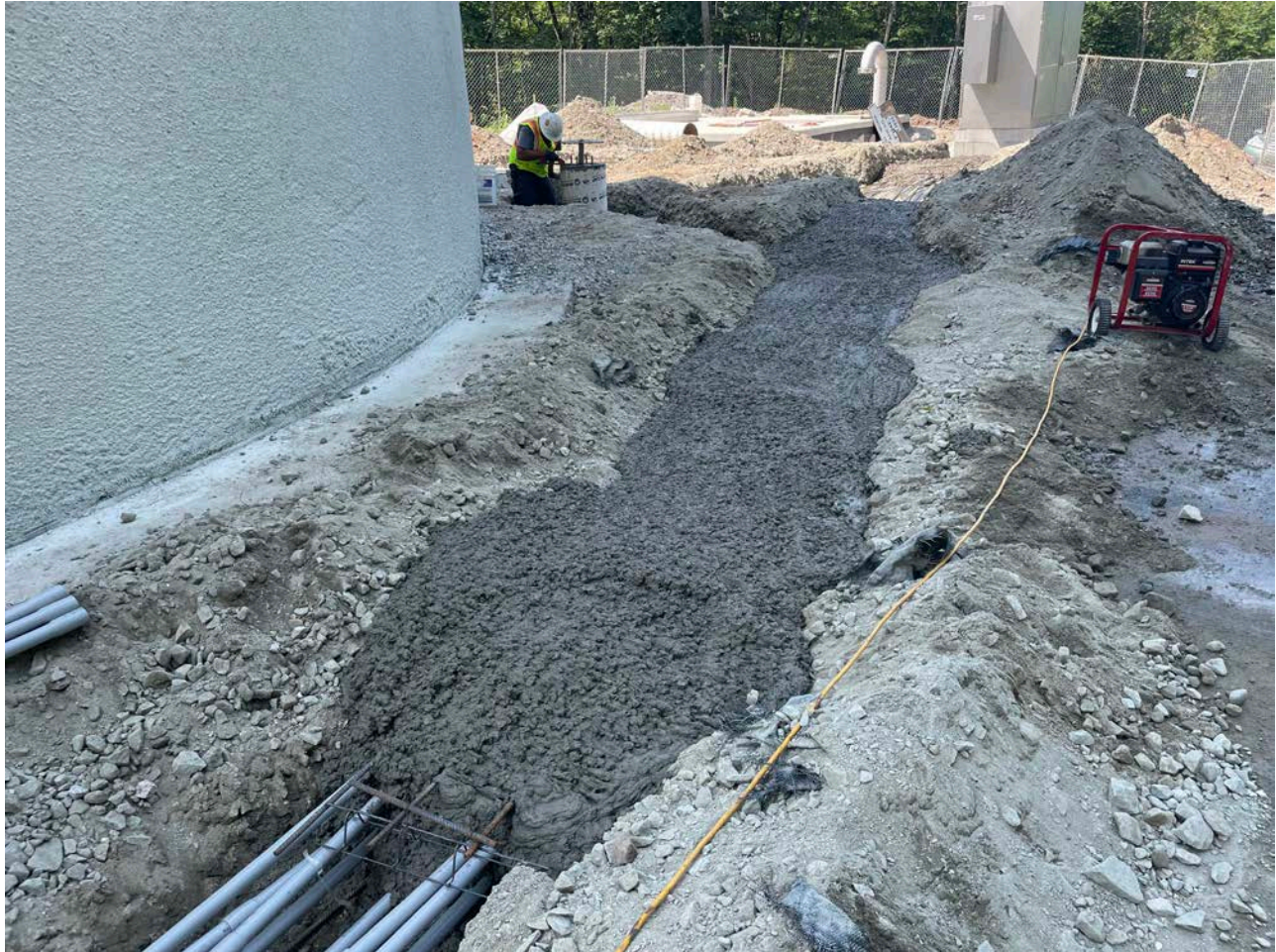
Picture 4: 4000 PSI concrete that was placed over sections of the utility duct bank today on the west side of the water tank located east of the Shared Access Driveway in Middletown. View to the south.
