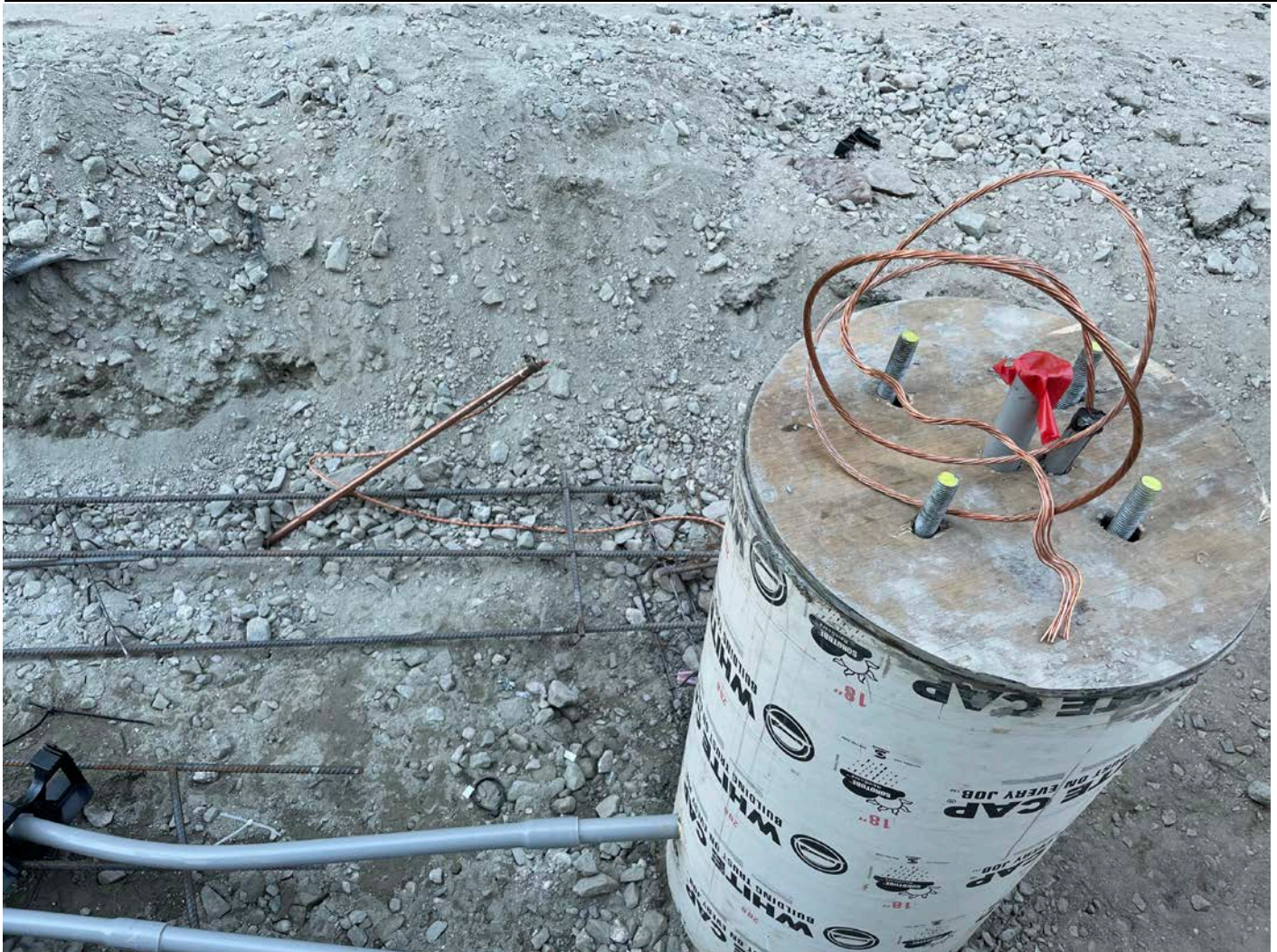
Picture 10: Ground line that A&R Electrical installed on the northeast side of the water tank located east of the Shared Access Driveway in Middletown.
