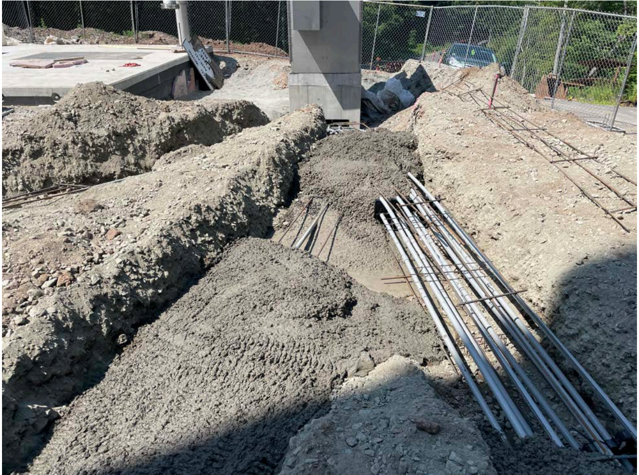
Picture 3: 4000 PSI concrete that was placed over sections of the utility duct bank today on the west side of the water tank located east of the Shared Access Driveway in Middletown. View to the west.
