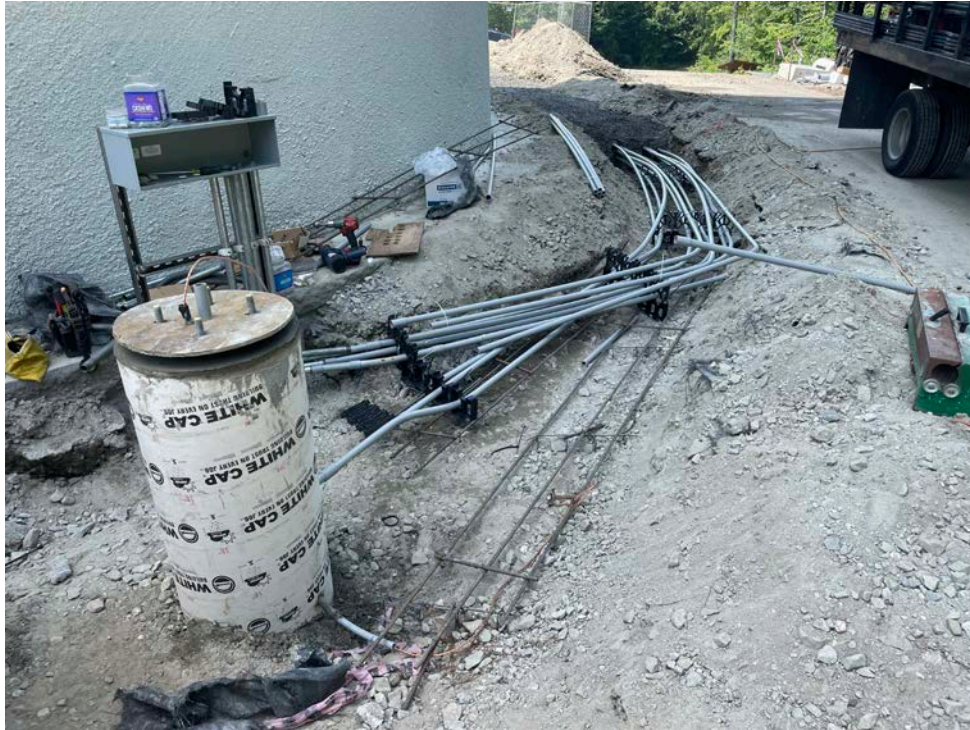
Picture 6: View of progress of the conduit installation on the north side of the water tank located east of the Shared Access Driveway in Middletown. View to the west.
