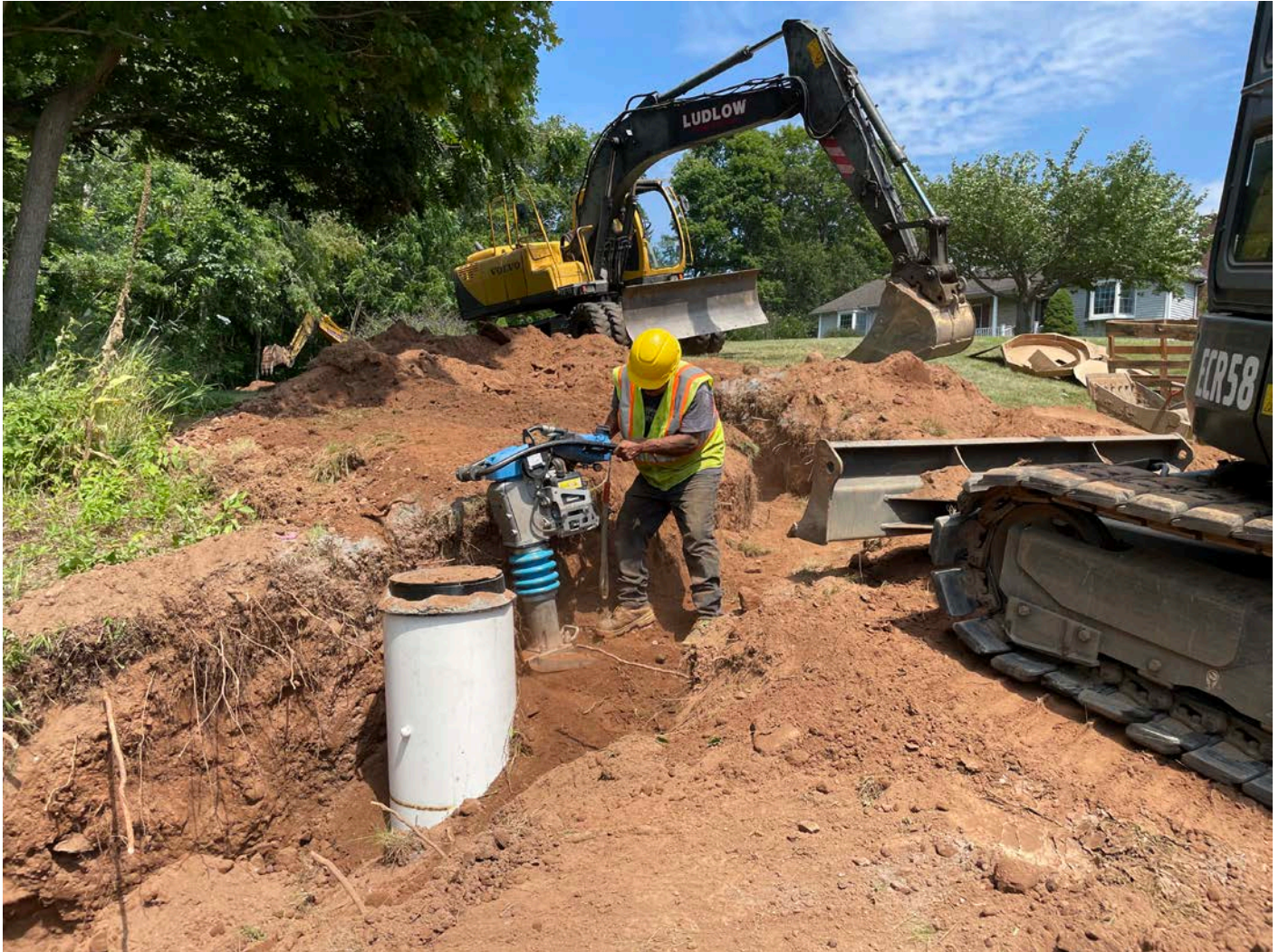
Picture 9: Ludlow compacting fill over 1.5" copper water service line they installed at the residence located at 10 Johns Way, Durham. View to the northeast.
