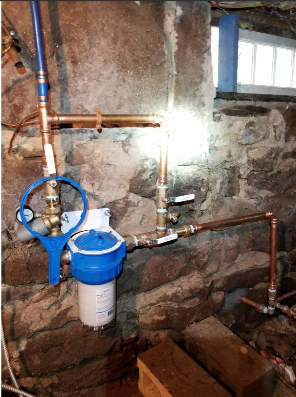
Picture 14: Final water service components that Fazzino Plumbing installed today at the residence located at 267 Main Street, Durham.
