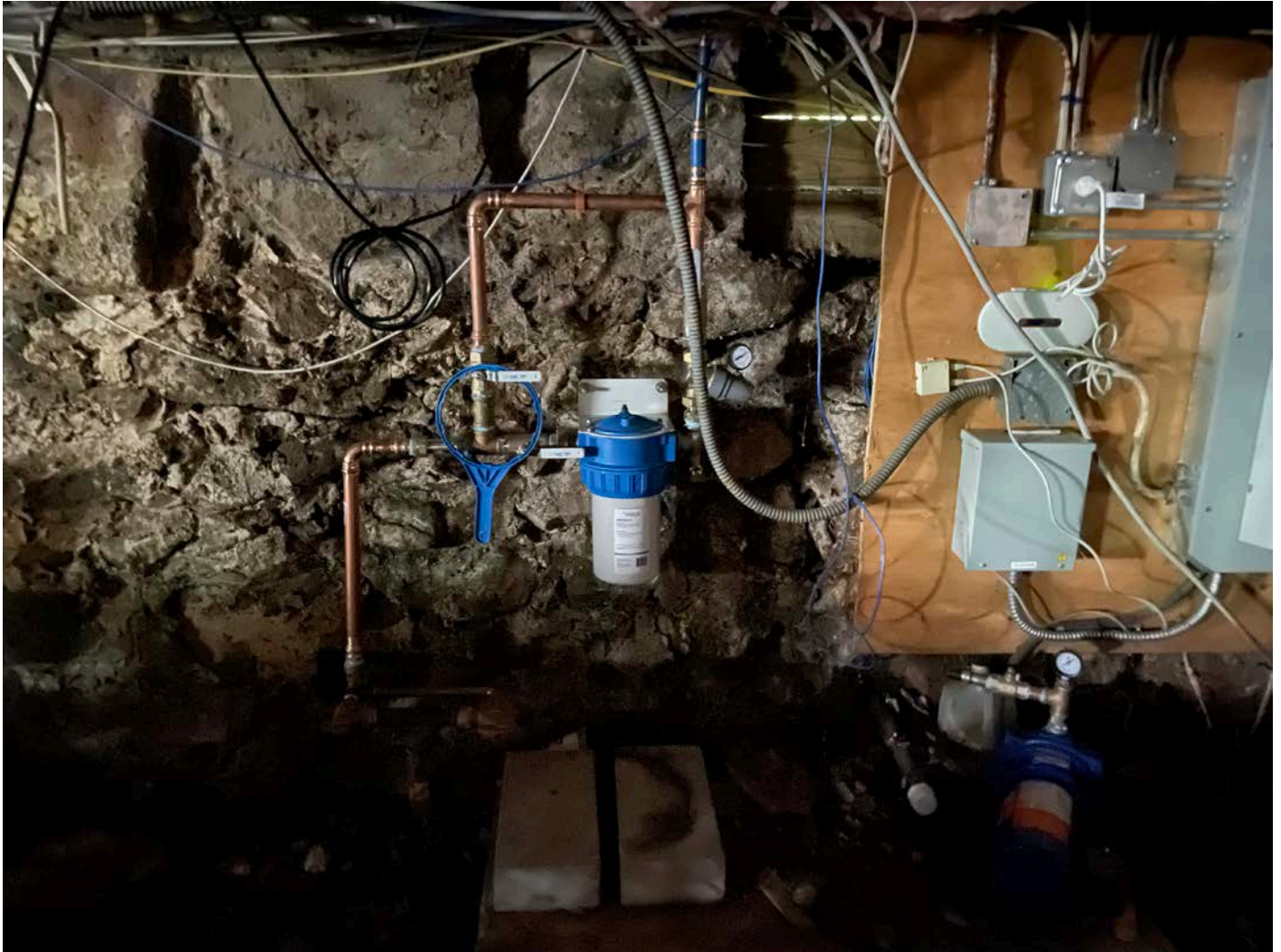
Picture 13: Final water service components that Fazzino Plumbing installed today at the residence located at 265 Main Street, Durham.
